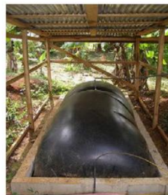
Fig. 3. Inflatable tubular digester (a) general scheme and (b) typical plant in Kenya.
