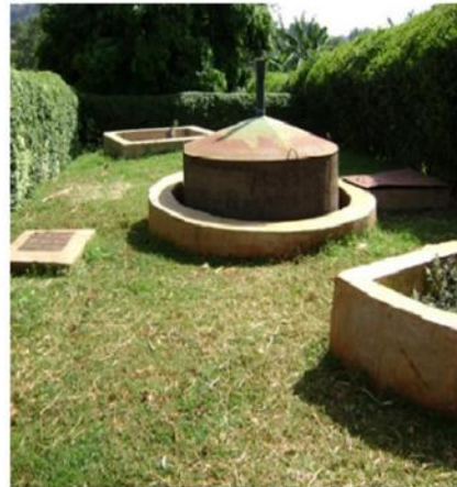
Fig. 1. Floating drum biogas digester: (a) general scheme and (b) typical plant in Kenya [30].
